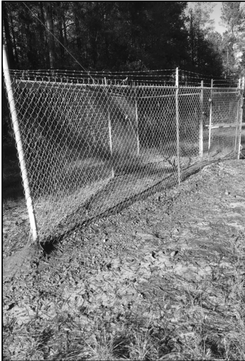
Guyed Tower Compound
